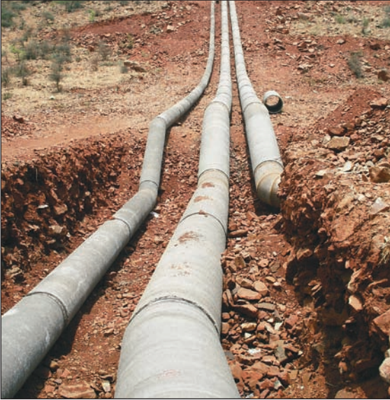
1000 mm & 600 mm dia M.S. Pipe lines for J. C. Nagi Reddy Drinking Water Supply Scheme, Phase II & III, Ananthapur District, Andhra Pradesh.
