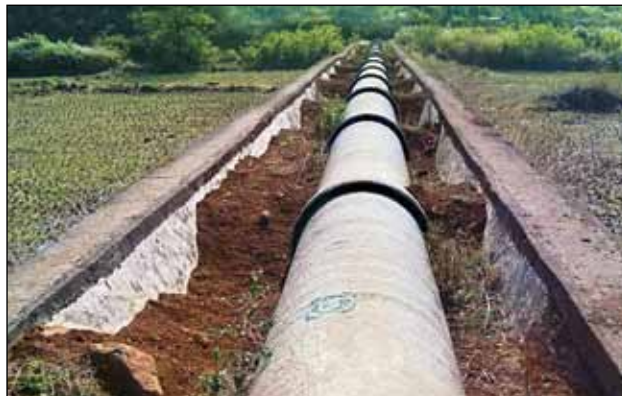
1100 mm dia PSC Pipe line for Vadiwale Left Bank Canal pipe line project Near Pune, Maharashtra
