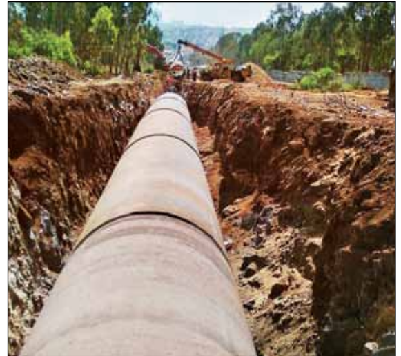
1825 mm dia duly lined & outcoated M. S. Pipe for W.S. Project Phase-II BWSSB-W5d Project Bangalore
