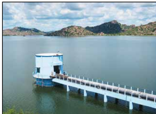
Intake well cum pump house for Mahabubnagar Water Supply Project, Hyderabad, A.P.
