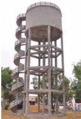
Elevated Service Reservoir of 1.3 Lakh Liter Capacity 16 Meters Staging for Palladam Water Supply Project
