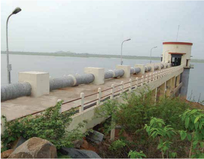
Intake Well cum Pump House
