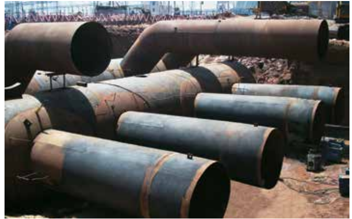
3750 mm dia x 1800 mm dia M.S. Pipes for Turbine Generator-2 at 2x600 mas D. B. Super Thermal Power Plant, Raipur
