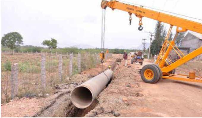
66.67 km, 900 mm dia MS pipes for Palladam Water Supply Project
