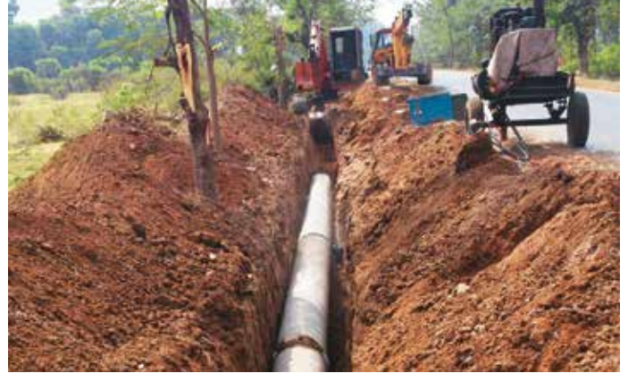
19.40 km, 400 mm dia BWSC pipes for Rajam Water Supply Scheme
