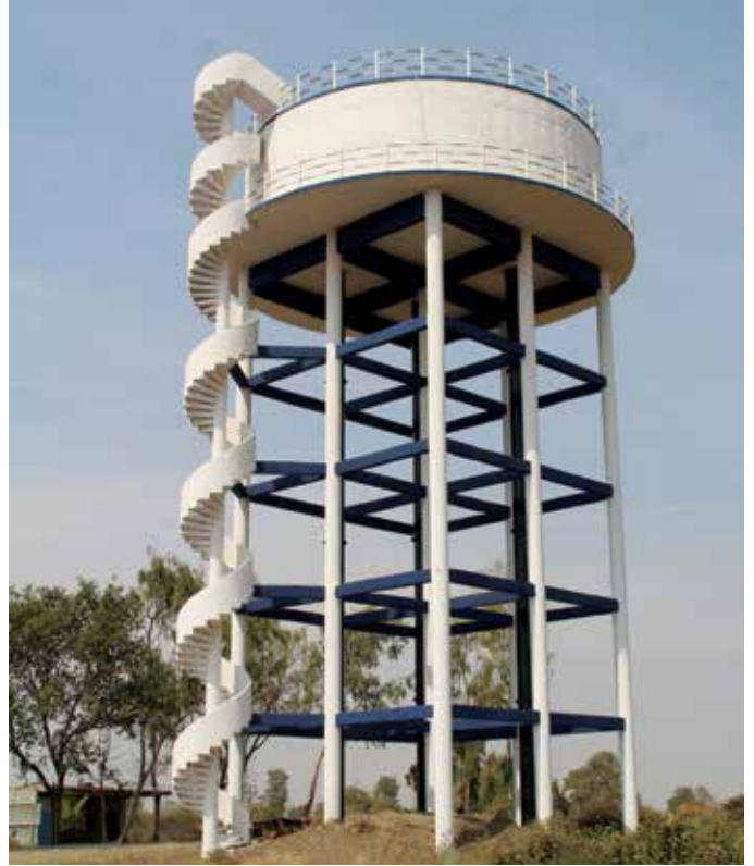
3.6 Lakhs Ltr Capacity Break Pressure Tank (BPT) at Buldhana Water Supply Scheme, in Maharashtra
