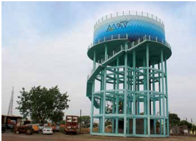
1000 KL Overhead Tank at Jora in Augmentation of Raipur Water Supply Scheme, in Chhattisgarh.
