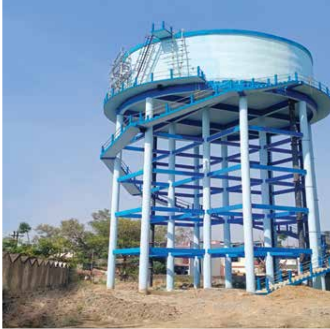
880 KL Overhead Tank staging 21 Mtr at Torwa for Bilaspur Water Supply Scheme, in Chhattisgarh
