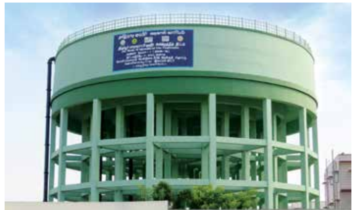
17.50 Lakh Litre Capacity Overhead Service Reservoir at Ishwargate for Tiruppur Water Supply Scheme, in Tamilnadu.
