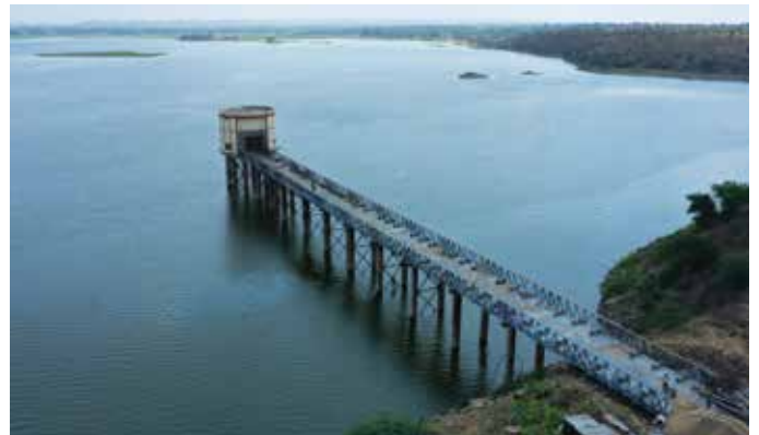
Intake well cum pump house - 13 mtr dia with Approach Bridge - 120 mtrs length x 6 mtr width based on Patadungrri dam for Hafeshwar Package-6 Project, in Gujarat
