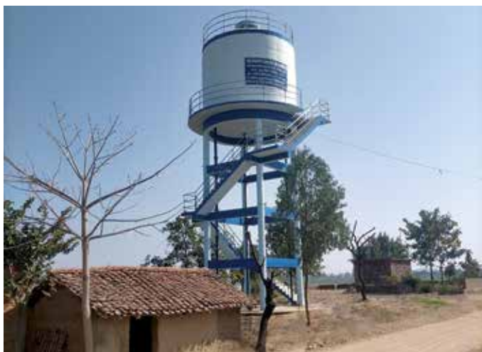
100 KL Overhead Service Reservoir at Chchp, Indwar Project in Madhya Pradesh
