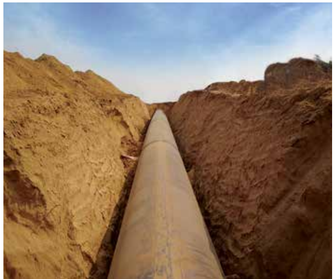
2028 mm dia outer diameter MS Pipeline laying at Tharad-Sipu Project, Palanpur Pkg-2, in Gujarat
