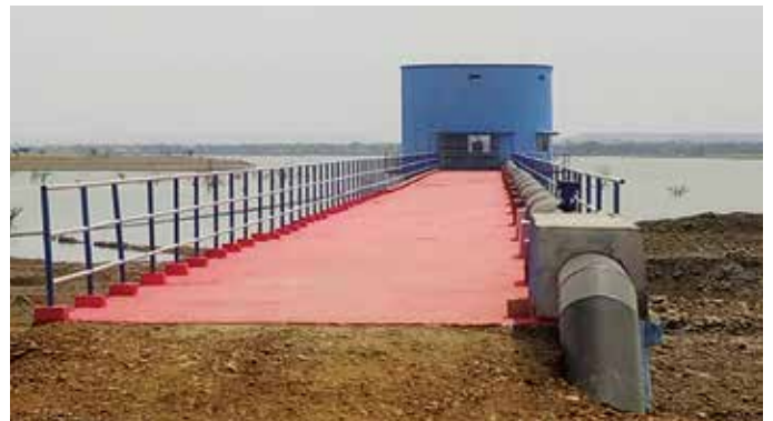
Intake Well, Approach Bridge and Raw Water Pumping Main at Bankpura Project, in Madhya Pradesh
